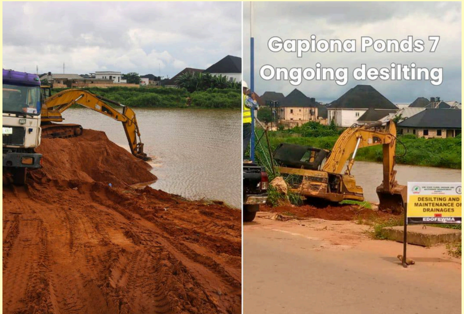
PHOTO CAPTION Ongoing desilting exercise at Gapiona in Benin City
